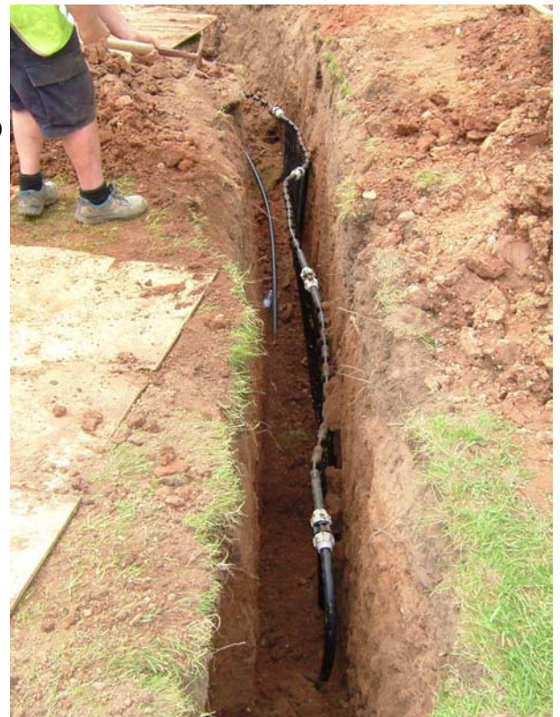
Vertical ground panels installed
