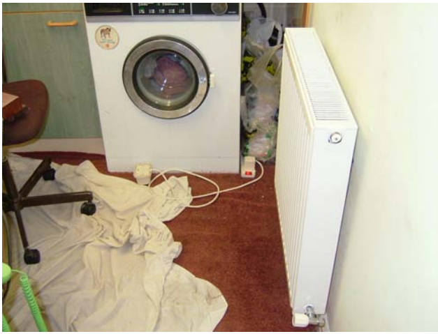
New radiator installed and working
