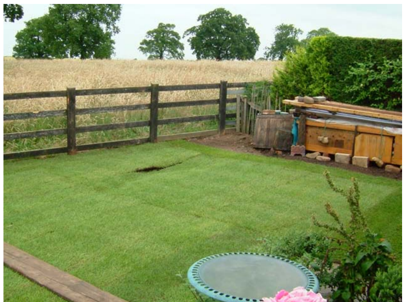
Post installation ground reinstatement completed and returned to lawn
