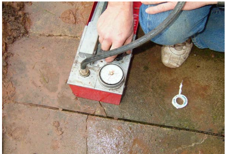
Pressure testing the ground loops
