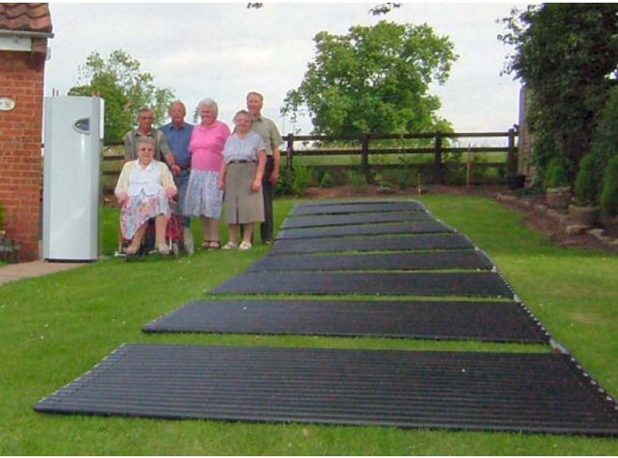
Ground panels laid out prior to ground work commencing
