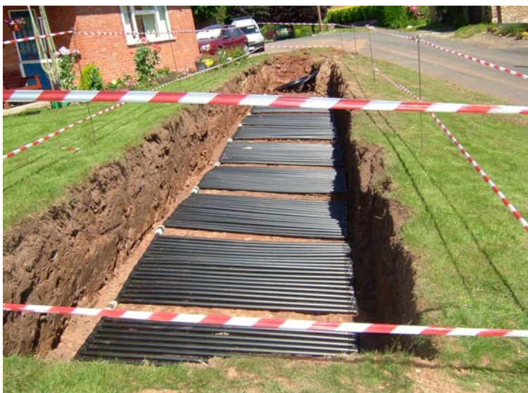
Nine panels laid horizontally and ready for back filling
