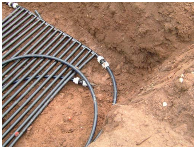
Connected ground panel in-situ
