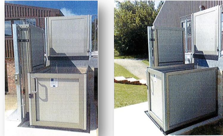
The new lifts in place at Great Ouseburn Village Hall.
