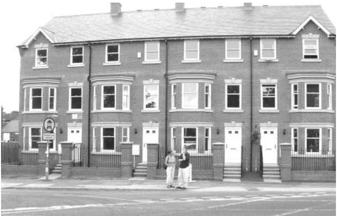
New housing under construction at former Ripon Land Rover site, Ripon
