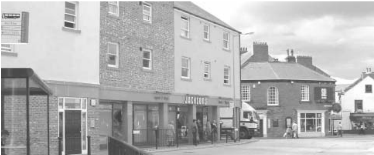
New retail unit as part of the redevelopment of Knaresborough Bus Station.
