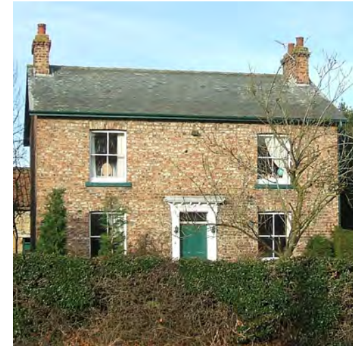
Ainsty Farm is constructed of traditional natural materials which are the most commonly used in the Conservation Area.
