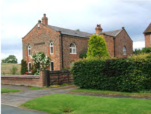
The former Wesleyan Chapel is evidence of the village's social history.
