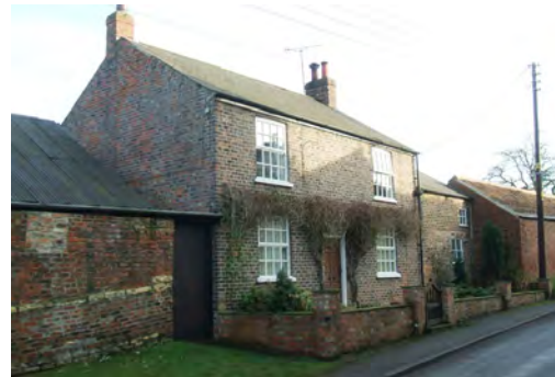
Village Farm is a good example of the simple, unadorned, but well proportioned building frontages found in Bilton in Ainsty.
