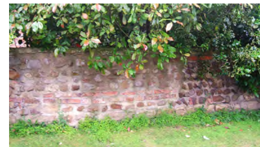
Three different boundary walls all on Church Street: The Old Chapel, Chestnut House and Ainsty Cottage respectively.
