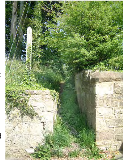
Public footpath alongside the Church wall
