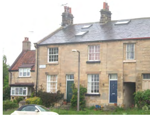
An example of ashlar limestone and rooflights.
