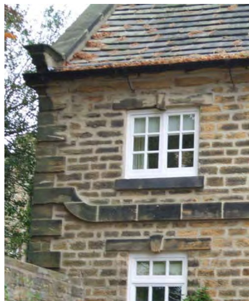
1st floor window and detail of the stonework inc. stringcourse, rusticated quoins, shaped kneelers and copings
