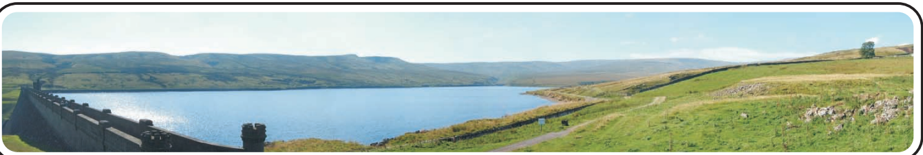
B Angram Reservoir and dam wall.
