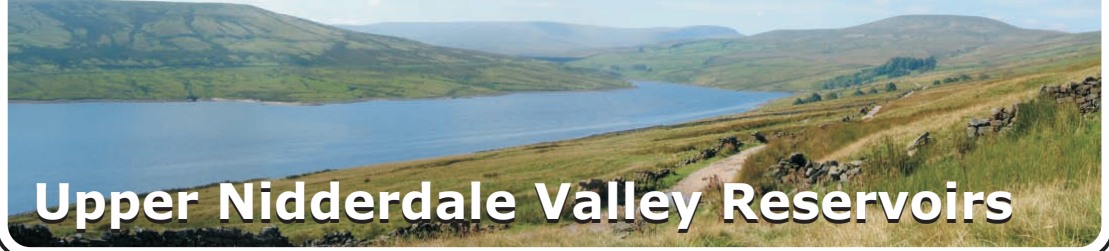
A Scar House Reservoir.
