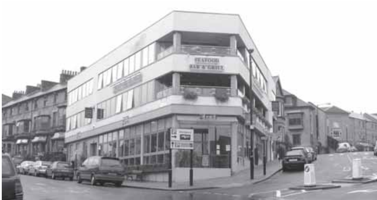
The recent facade to Town Centre House, Cheltenham Crescent/Parade, Harrogate .
