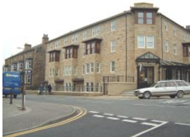
A derelict night club site has been redeveloped to provide affordable housing and retailing in Harrogate town centre.
