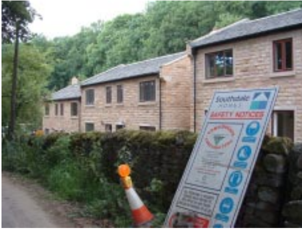
New affordable housing built recently in Fewston.
