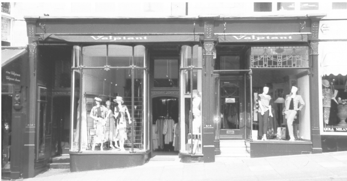
50/52 Parliament Street, Harrogate: an Edwardian shopfront incorporating many typical features.
