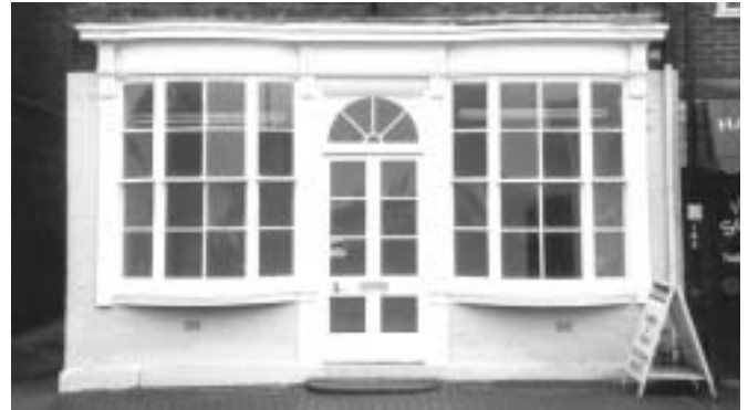
14 High Street, Knaresborough: a recently restored early C19 shopfront
