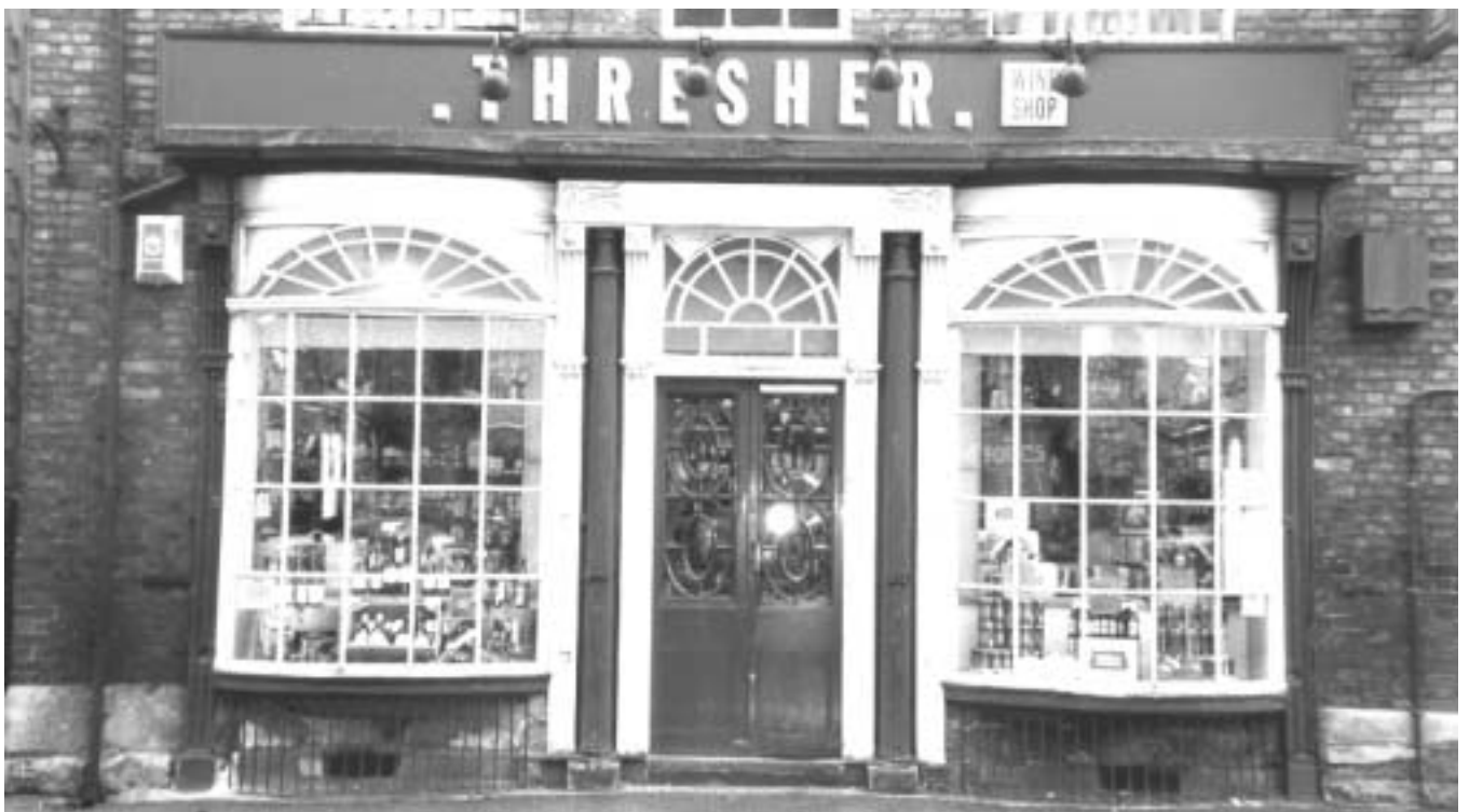
48 High Street, Knaresborough: one of the finest shopfronts in the District, although somewhat spoilt by the advertising board above the cornice.
