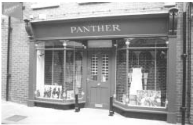
A well-proportioned "new traditional" shopfront with discreet signage
