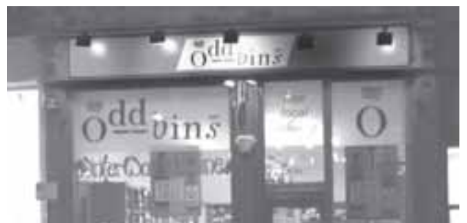
Externally illuminated fascia.
