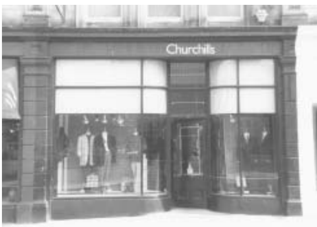
Simple signage to an Edwardian shopfront
