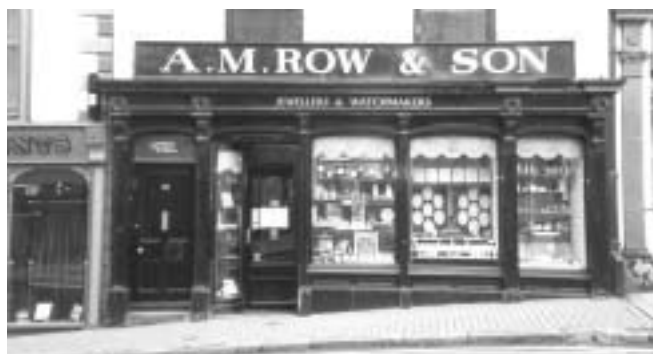
Victorian: full height panes divided by pilasters with consoles supporting the entablature
