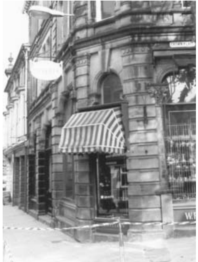
a poorly designed canopy, unrelated to the building
