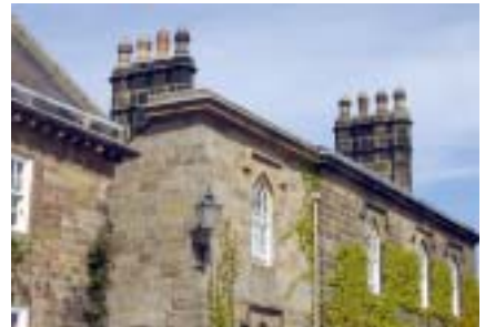
Well-designed, early 1990's extension to the Boar's Head.
