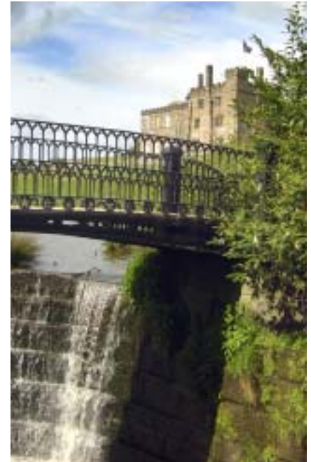
Weir and footbridge over Ripley Beck, Hollybank Lane.
