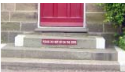
An inappropriate notice on a doorstep in the Market Place.
