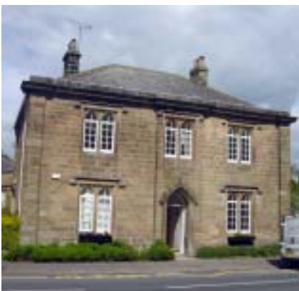
School House, Main Street.
