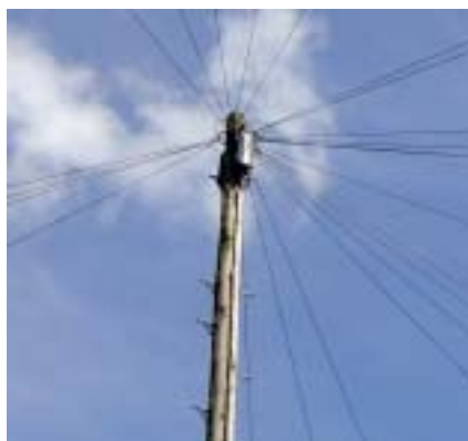
Overhead cables are a visual detractor.
