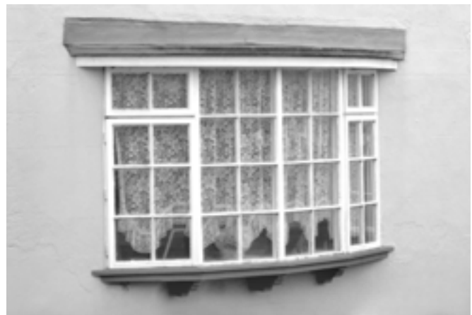
A mock-Georgian bay has replaced the original vertical sliding sash window - to the detriment of the facade.
