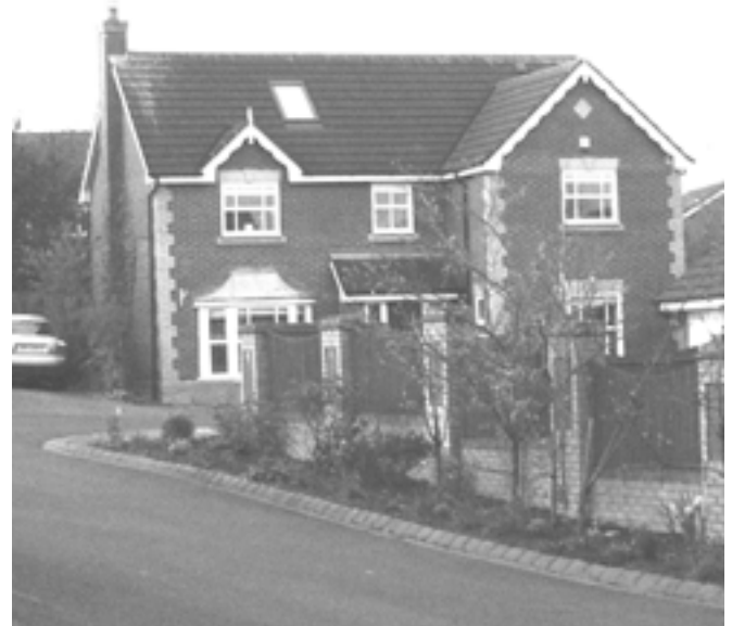
Two rooflights on opposite slopes of the roof resulting in an apparent 'hole' in the roof.
