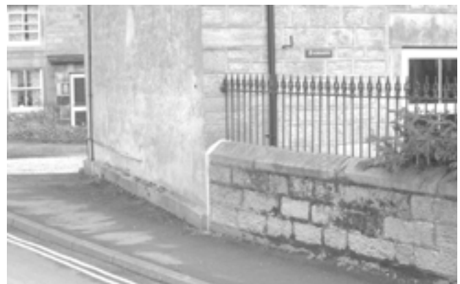
Iron railings lead into stone coping.
