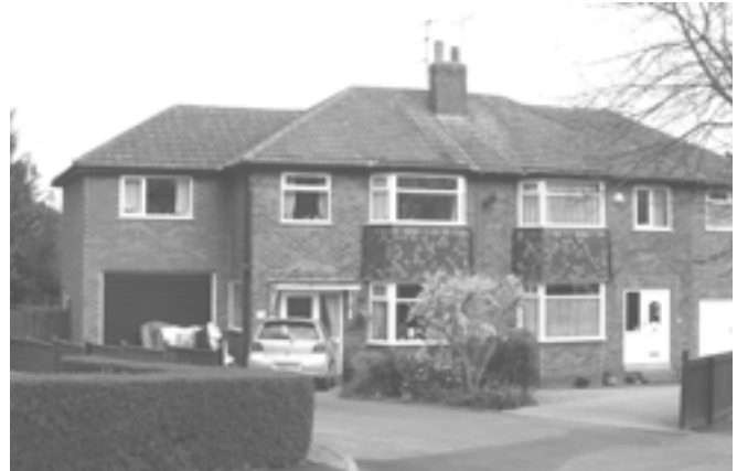
Extension set well back and reflecting the original form of the house.
