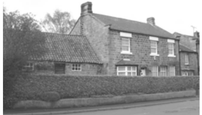
Outbuilding with pantiled roof against house with a slate roof.
