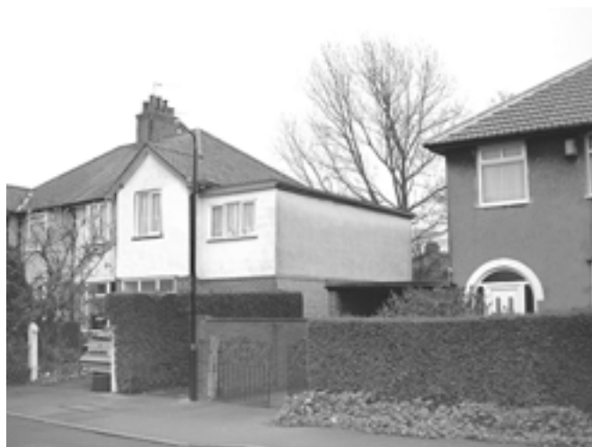
Prominent flat-roofed extension is visually detrimental.
