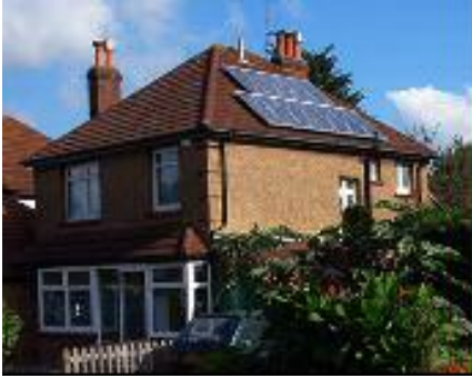
Domestic Solar PV system
